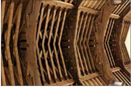
11. Scissor-braced Roof
